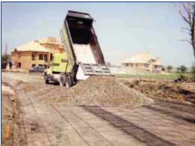
Photo 1: Back dump spread over geogrids
