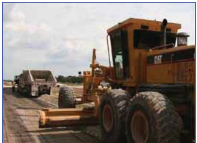
Photo 2: Belly dump spread over geogrids
